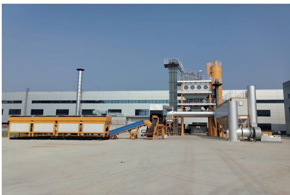
LB Asphalt Batch Mixing Plant in Nigeria
