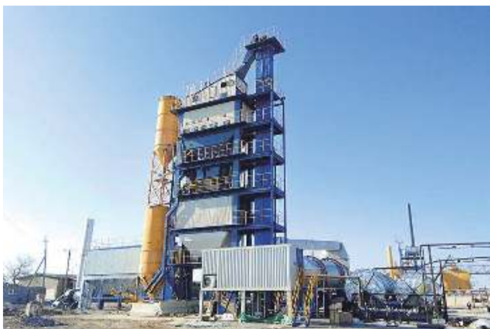
240TPH Asphalt Batch Mix Plant Running Smoothly in Uzbekistan
