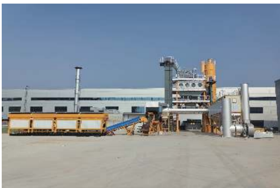
LB Asphalt Batch Mixing Plant in Nigeria
