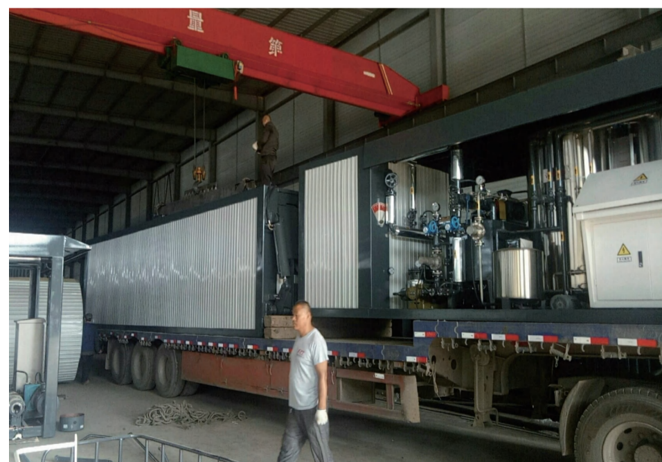
Bitumen Emulsion Plant in Africa Cairo, Africa, treated 300 tons of asphalt to build roads April 21th, 2019
