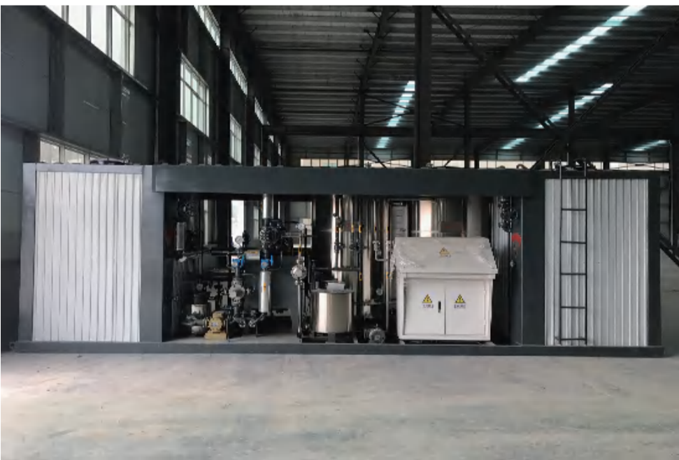
Bitumen Emulsion Plant in Ethiopia Addis ababa, Ethiopia, treated 200 tons of asphalt for road construction November 27th, 2019
